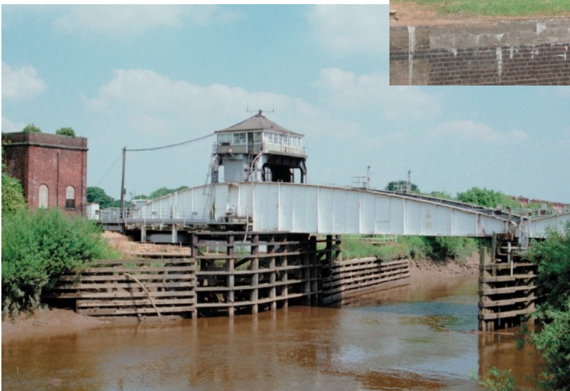
The railway bridge over the Ouse at Selby.
