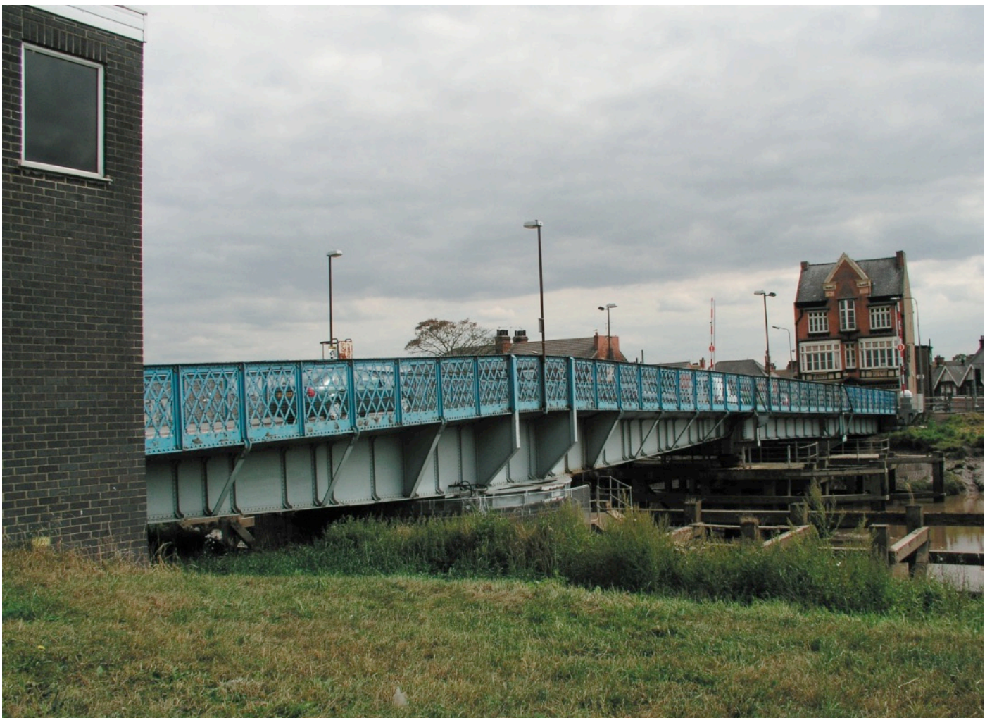
The bridge from the northern bank.
