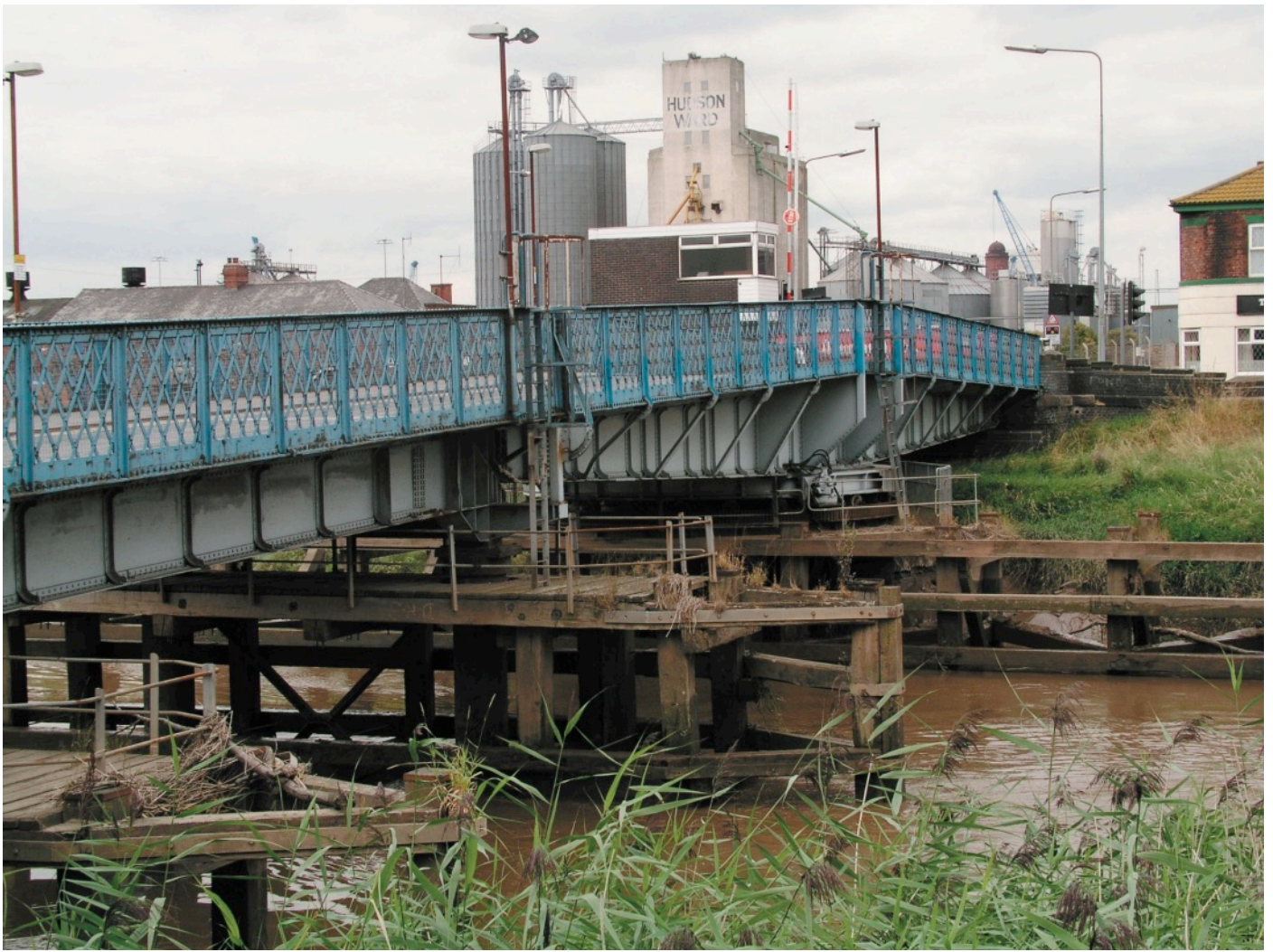
The bridge from the south east.
