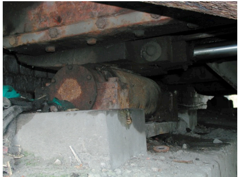
Below, details of the bridge wedge and north abutment.
